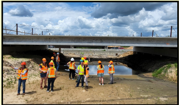
Dr. Jennifer Korn (FLTWS Newsletter Editor), Nicole Monies (FDOT), Amber Crooks (Conservancy of Southwest Florida), and others, tour the new wildlife crossing currently under construction on I-4.
